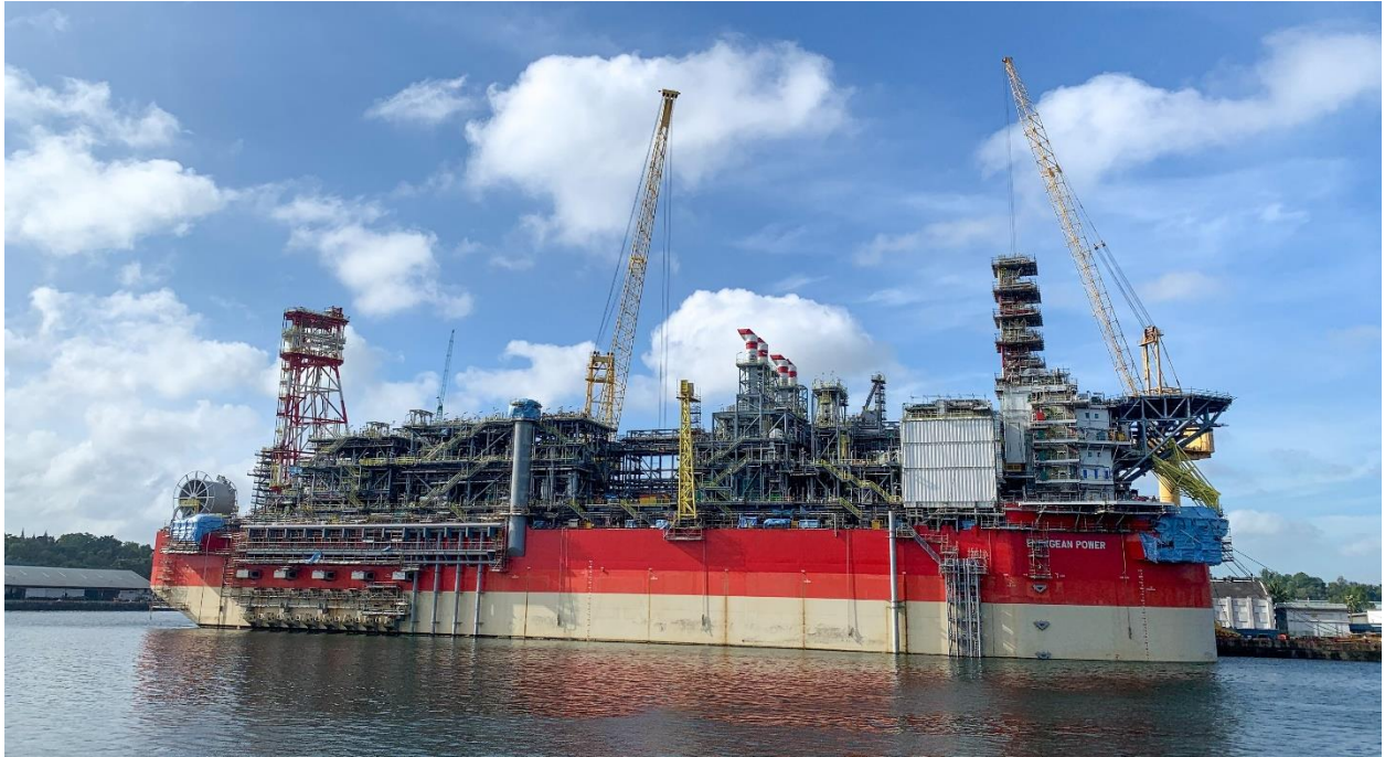
Fig. 3 – The Energean Power FPSO in Singapore
