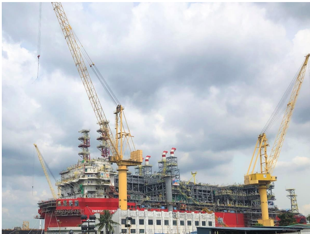
The Energean Power FPSO at the Admiralty Yard, Singapore
